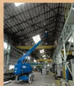
LED 設置工事
